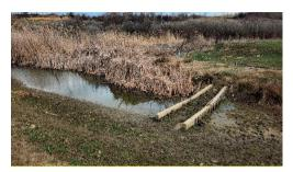
Figure 10. Blockage of the drain channel (13.03.2025)
