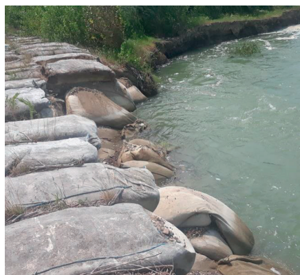
Figure 18. Degradation of geocontainer works by lowering the elevation of the riverbed and relocating the geocontainer, Siret river, Suraia locality, Vrancea county (photo taken by the authors)
