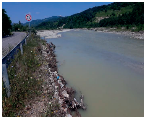
Figure 15. Gabion works of 300 m length degraded by floats, Zabala river, Naruja locality, Vrancea county (photo taken by the authors)
