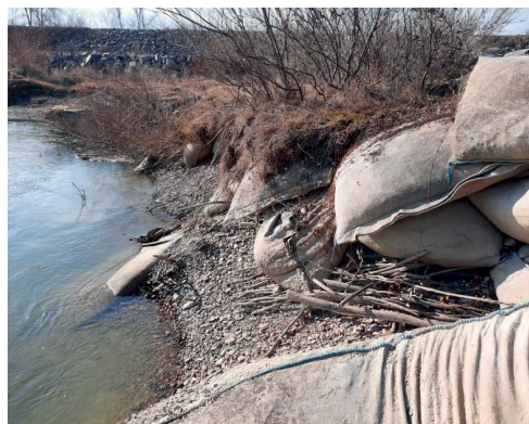
Figure 16. Degradation of geocontainer works by reducing the riverbed quota, Siret river (photo taken by the authors)
