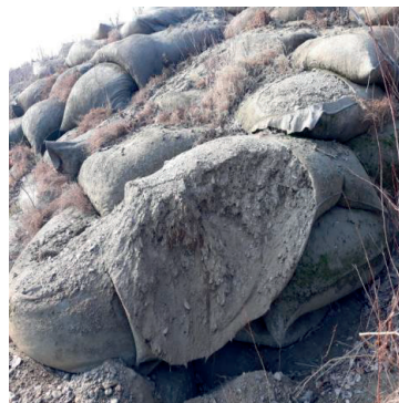
Figure 19. Geocontainer works degraded by vandalism, Siret river, Vadu Rosca, Vrancea county (photo take by the authors)
