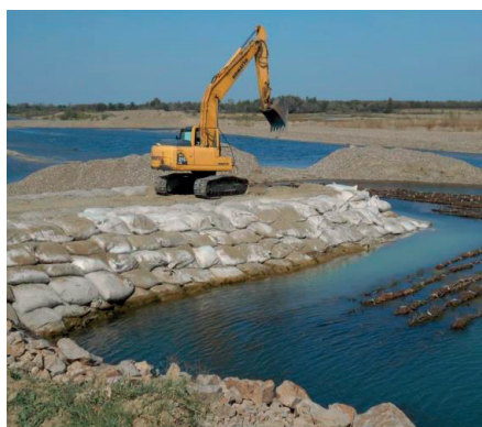
Figure 5. Geocontainer work in the form of haulers, 500 m length on Siret river, Suraia locality, Vrancea county (photo taken by the authors)
