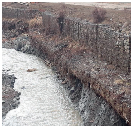
Figure 14. Gabion works of 200 m length degraded by the decrease of riverbed quota, Coza river, Tulnici, Vrancea county (photo taken by the authors)
