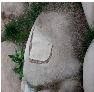
Figure 19. Geocontainer works degraded by vandalism, Siret river, Vadu Rosca, Vrancea county (photo take by the authors)
