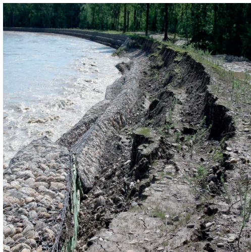
Figure 13. Gabion works of 2700 m length degraded by slip Putna river, Vidra locality, Vrancea county, Q = 670 \text{ m}^3/\text{s} (photo taken by the authors)
