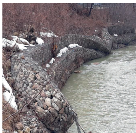
Figure 12. Gabion works of 300 m length, degraded by overturning, Putna river, Tulnici city, Vrancea county, Q=570 \text{ m}^3/\text{s} (photo taken by authors)
