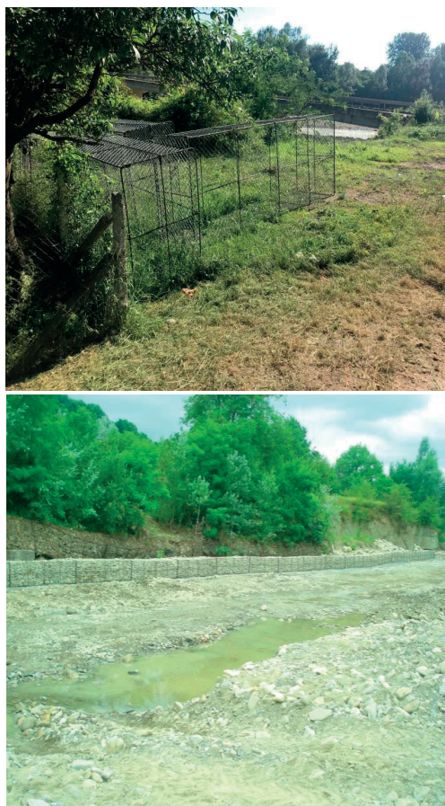
Figure 1. Classic gabion work, 200 m length, on Putna river in the village of Valea Sarii, Vrancea county (photo taken by the authors)
