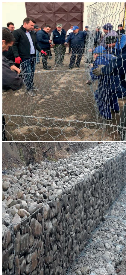
Figure 2. Alternative gabions work, 450 m with a length on Oreavu stream, Urechești locality, Vrancea county (photo taken by the authors)
