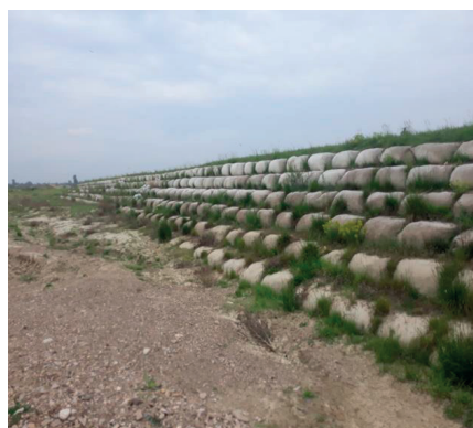
Figure 6. Longitudinal geocontainer work, 240 m length, Ramnicu Sarat river, Ramnicu Sarat locality, Buzau county (photo taken by the authors)
