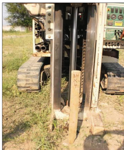
Figure 5. Drilling of BH4
