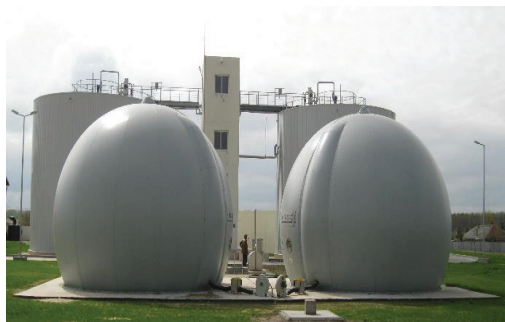
Figure 6. Methane tanks and fermenters for sludge processing
