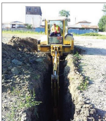
Figure 4. Digging of TP26
