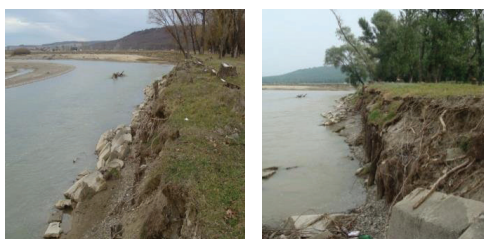
Figure 6. Degradation of left shore protection works of Moldova River after floods in 2010
