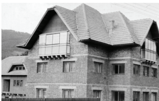
Figure 12. City type rural three storied brick masonry dwelling with RC floor slabs and without RC belts
