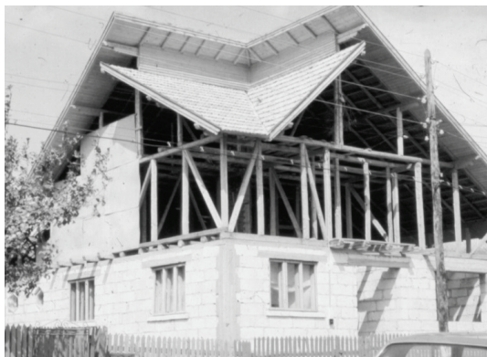
Figure 7. A traditional dwelling with roof band and RC lintels, pillars at corners, a light roof, in 2-4 slopes having a structure well tight with the masonry
