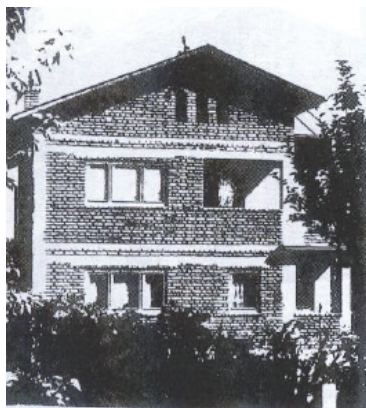
Figure 3. City type rural two storied brick masonry dwelling with embedded RC columns and RC slabs (the collar beam as a frame beam)
