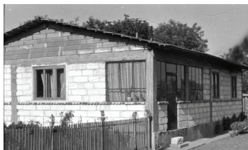
Figure 10. A traditional dwelling with RC floor slabs (lintels are embedded in RC floor slab)
